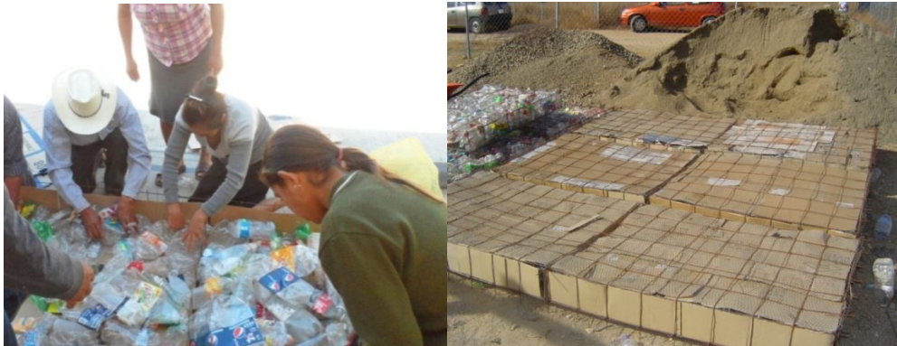
Figure10. Women and men filling the panel with recycled material. (Photos: J. Caballero, 2010)
