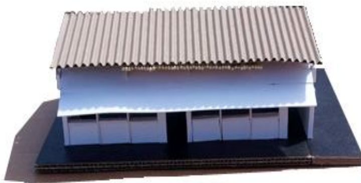
Figure 7. Bioclimatic strategies-second roof on classrooms. (Photo: R. Alavéz)
