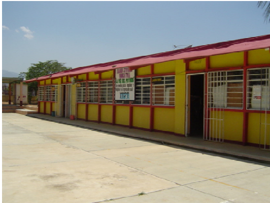
Figure 2. School built with ferrocement technology. Sta. María Roaló, Zaachila. (Photo: J. Caballero, 2010)
