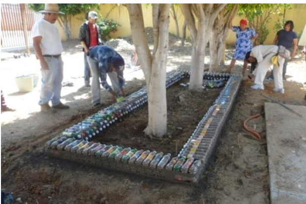
Figure 9. Construction of planters using plastic bottles. (Photo: J. Caballero, 2010)
